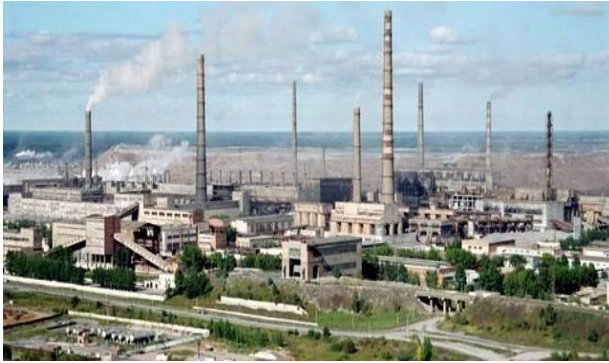
Achinsk Alumina Refinery
